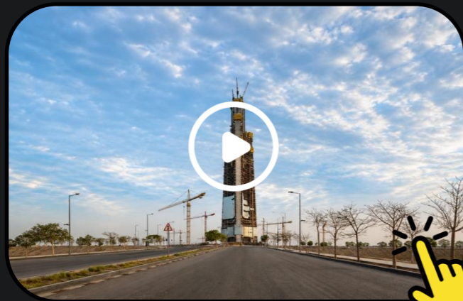
Jeddah Tower 100 Floors
