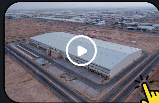
Al-Shaya Mega Warehouse
