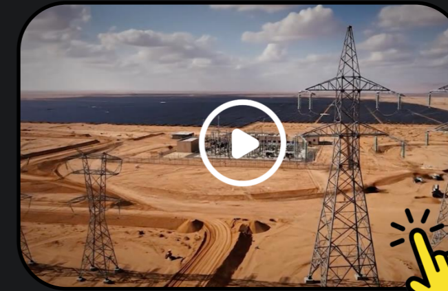
AlSaad EV Power Plant
